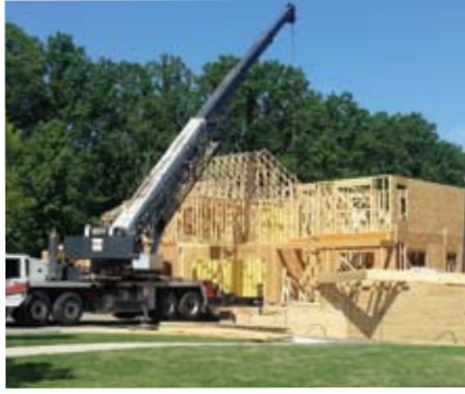
Hoisting Roof Trusses for New Villas
