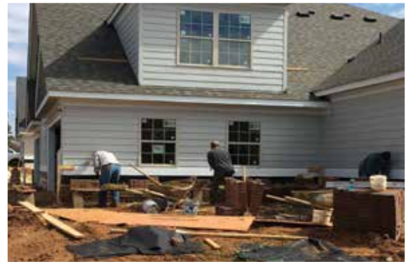
Installing brick accents
