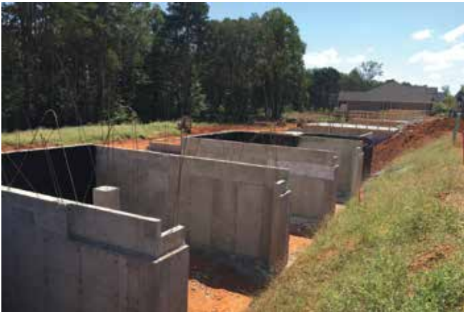
Big Creek - Basements Lined Up for Construction
